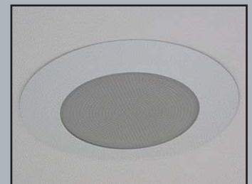
Sealed Recessed Light in Wet Areas
