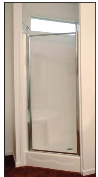
49" Corner Shower - Replacing Corner Soaker Tub & Adding Linen Closet in place of Original Shower
