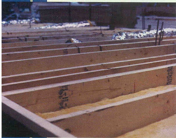
Floor joist construction is completed under optimal conditions and quality control within this Commodore factory.
